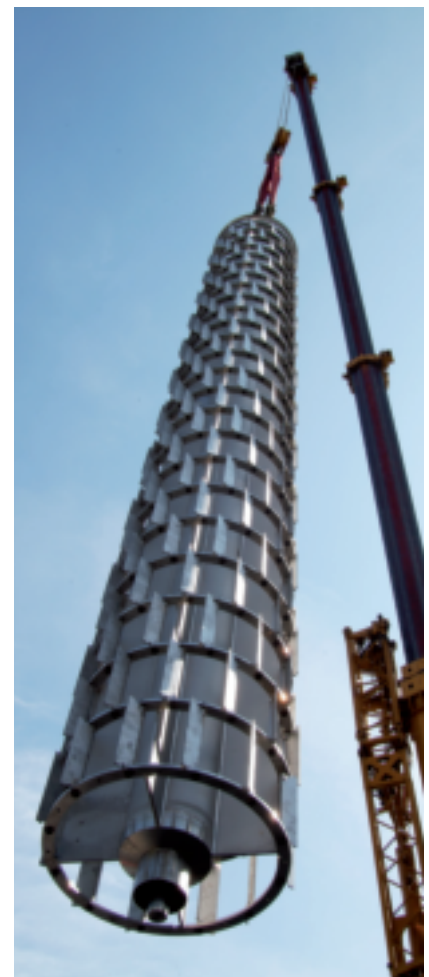
On-site installation of a rotor into a wiped film evaporator
