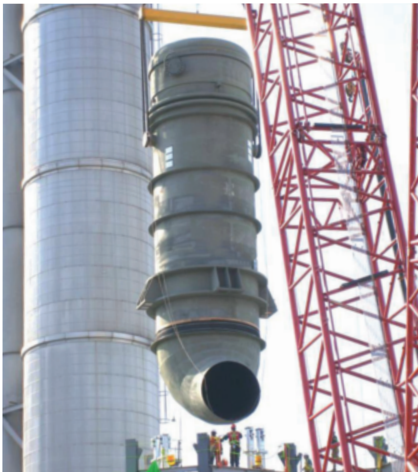
On-site installation of a large falling film evaporator
