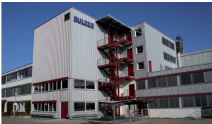
Sulzer test center in Allschwil, Switzerland
