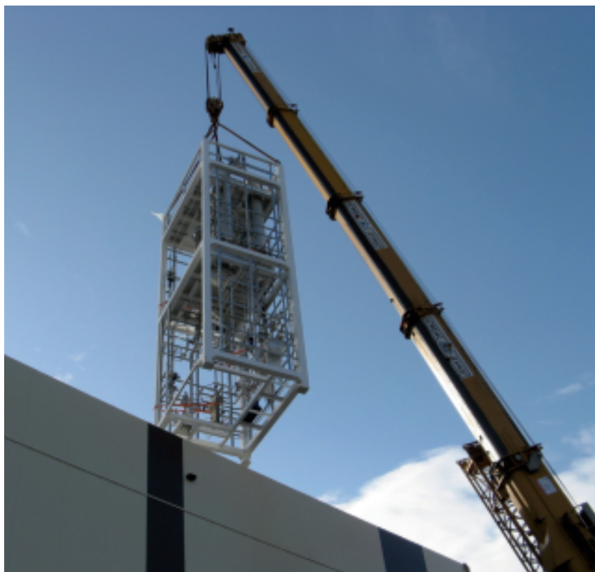
Two-stage skid-mounted evaporation unit with a falling film evaporator and a wiped film evaporator
