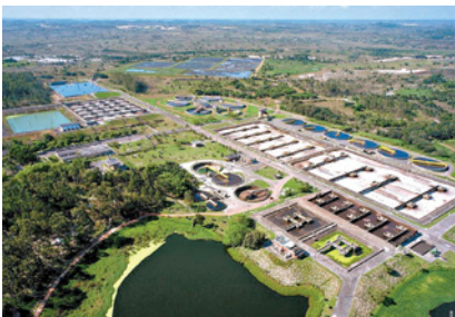
Cetrel industrial wastewater treatment plant in Camaçari/Bahia-Brazil
