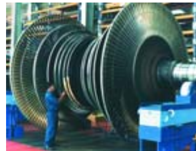
2 Re-blading work on a 56-ton low-pressure steam turbine rotor.
