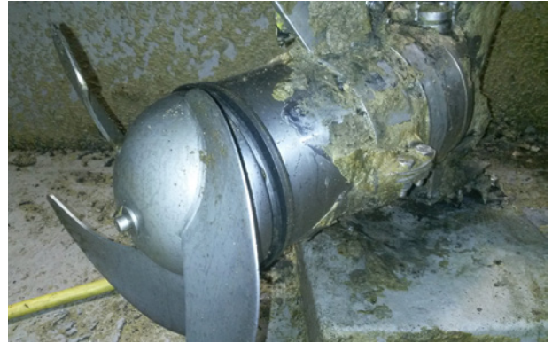
Mixer inspection after six months of operation
