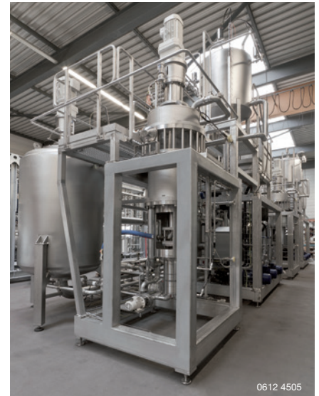
Industrial freeze concentration unit
