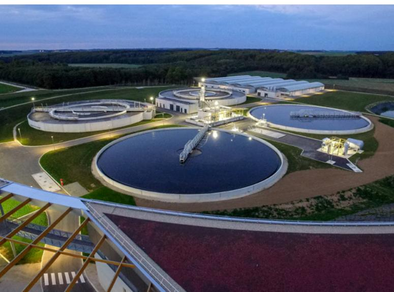
Launched in 2017, the Chartres Métropole conurbation wastewater treatment plant in Mainvilliers (28) has twice the capacity of the old plant at Lèves. This new installation, which today receives wastewater from the conurbation's twelve municipalities, operates with a capacity of 160'000 population equivalents, with the possibility to be adjusted as the area develops and the potential to increase treatment capacity by a further 25%.
