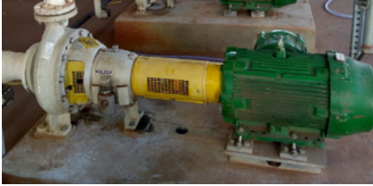
SNS3-80 pumping unit for anhydrous ethanol
