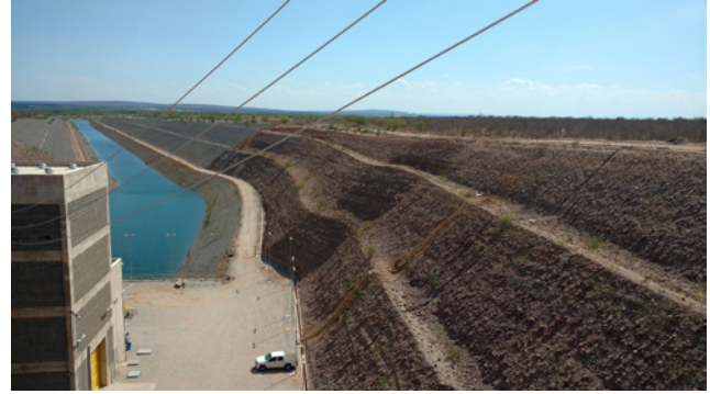
The pumps deliver water into a network of canals that has been 10 years in the planning
