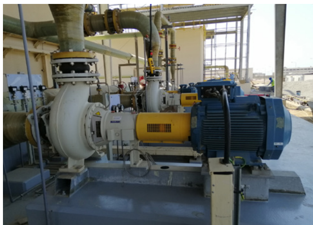
Each site uses a selection of Sulzer pumps, including the AHLSTAR single-stage centrifugal process pump and MBN-RO high pressure pump.
