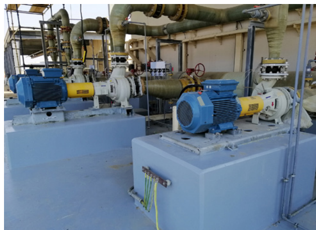
Each site uses a selection of Sulzer pumps, including the AHLSTAR single-stage centrifugal process pump and MBN-RO high pressure pump.
