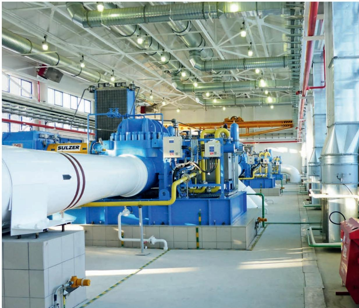
7 Pumping station of the ESPO pipeline with Sulzer pumps in operation.
