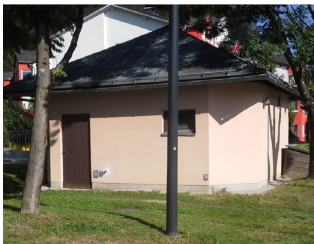
Network pumping station in Zell am See
