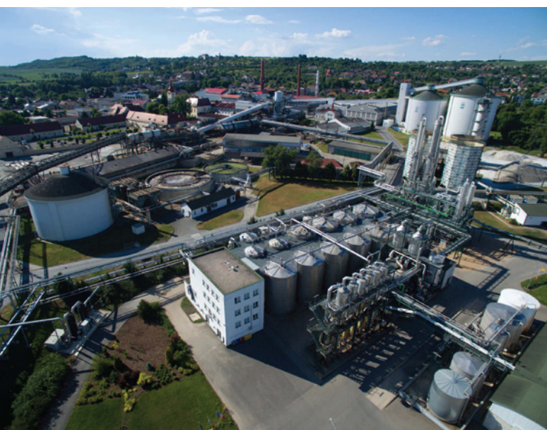
The Tereos Dobrovice plant with an integrated WWTP
