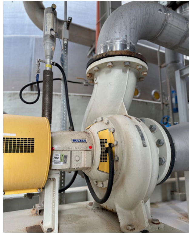
AHLSTAR APP43-300 pump with SP8 seal pot for beer
