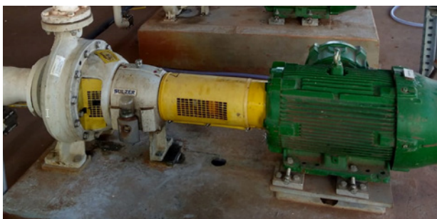
SNS3-80 pumping unit for anhydrous ethanol
