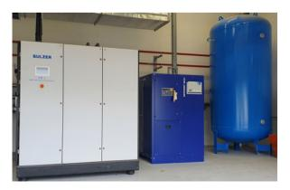
Traditional designs of compressor suffer from increased levels of wear over the years, and with five-figure bills commonly attributed to annual maintenance, a performance review of the compressed air system could yield significant savings. For example, Sulzer's development of the HSR oil-free turbocompressor product line uses active magnetic bearing technology, eliminating any lubricated bearings or seals and offers a near maintenance-free machine.
