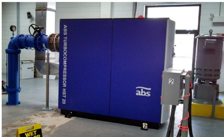
HST 20 turbocompressor installation at the wastewater treatment plant of Neptune
