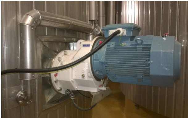
SALOMIX SLF-80.18DG side-mounted horizontal agitator on wheat glucose syrup storage tank
