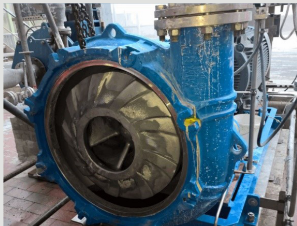
Figure 5. EMW pump during inspection
