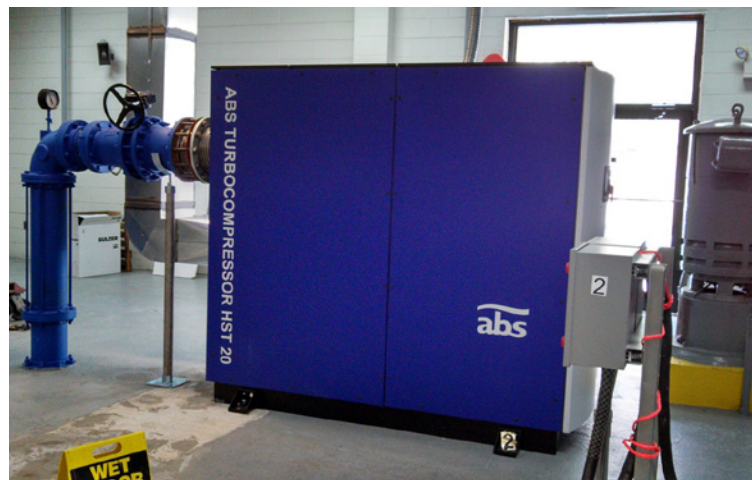
HST 20 turbocompressor installation at the wastewater treatment plant of Neptune
