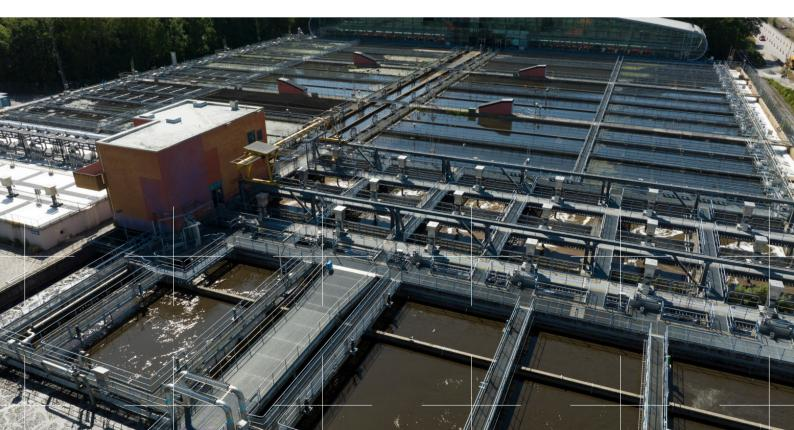
The Gryyab wastewater treatment plant handles all the effluent from the greater Gothenburg area, the second largest city in Sweden. Its state-of-the-art design minimizes energy consumption, with advanced treatment processes removing waste and converting it to organic soil enhancer or using it to contribute to the local district heating system.
