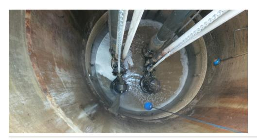
View from the top of the well. Particularly arduous as the inflow falls directly on top of the pump.
