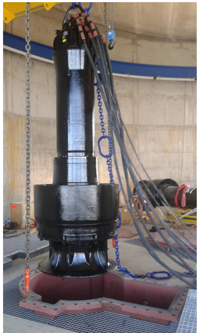
AFLX about to be lowered into riser pipe.
