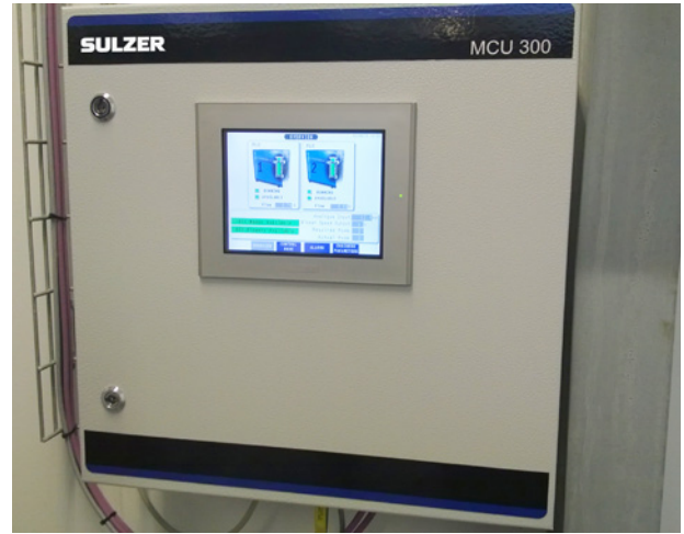
The master control unit in the compressor room
