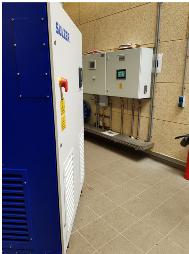
The MCU is connected to a pressure sensor and ensures efficient control of the turbocompressors.
