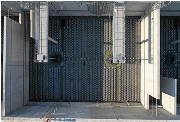
Today's state-of-the-art solution for municipal wastewater aeration is the membrane disc. Pictured here are Sulzer disc diffusers delivered to Europe's largest wastewater treatment plant (Vienna, Austria).
