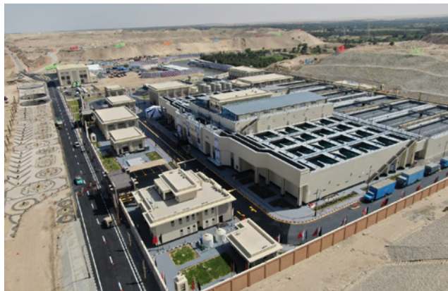
The construction project delivered a reliable and efficient plant, with a minimal footprint, capable of achieving low operating costs (Image source: Metito)
