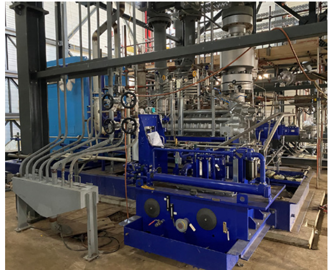
Site installation of feedwater pump
