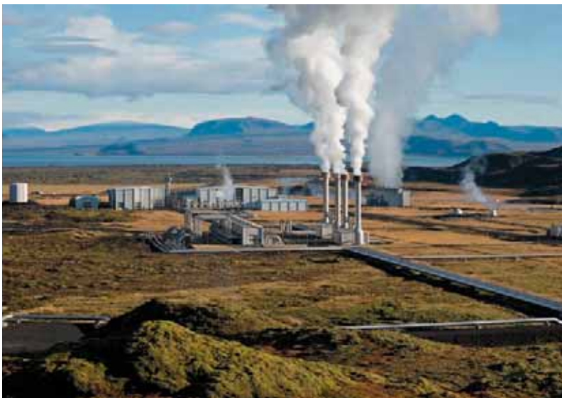
4 Nesjavellir geothermal power plant in Iceland.
