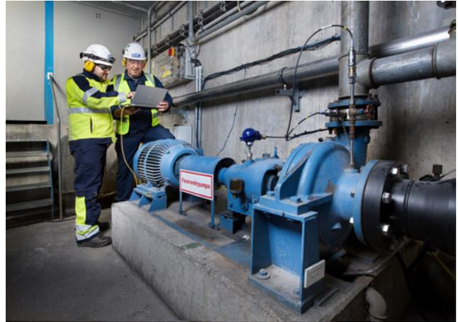
Diagnosed after DOC BOX installation: The pump is running outside its performance range
