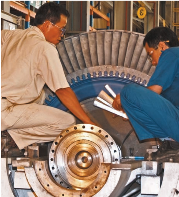
4 Reassembly of the turbine at the shop.
