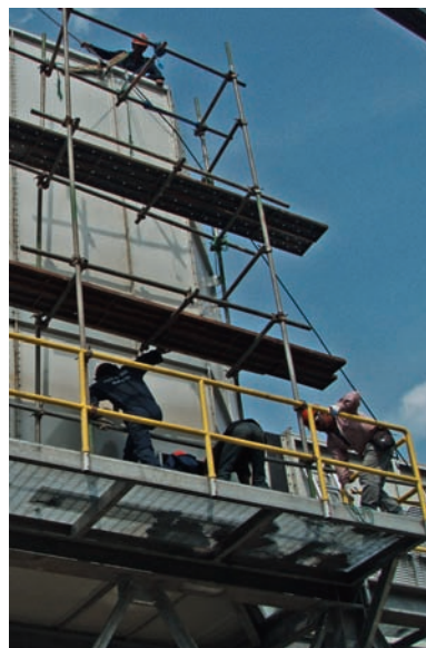
⑧ The inlet air system was reassembled on-site.
