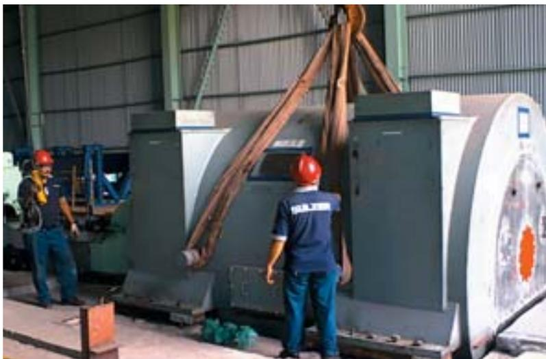
**1** Sulzer Turbo Services reconditioned and installed 2 turbine generator units that provide additional energy for a pulp mill on Sumatra, Indonesia. This image shows the setting of the generator casing.
