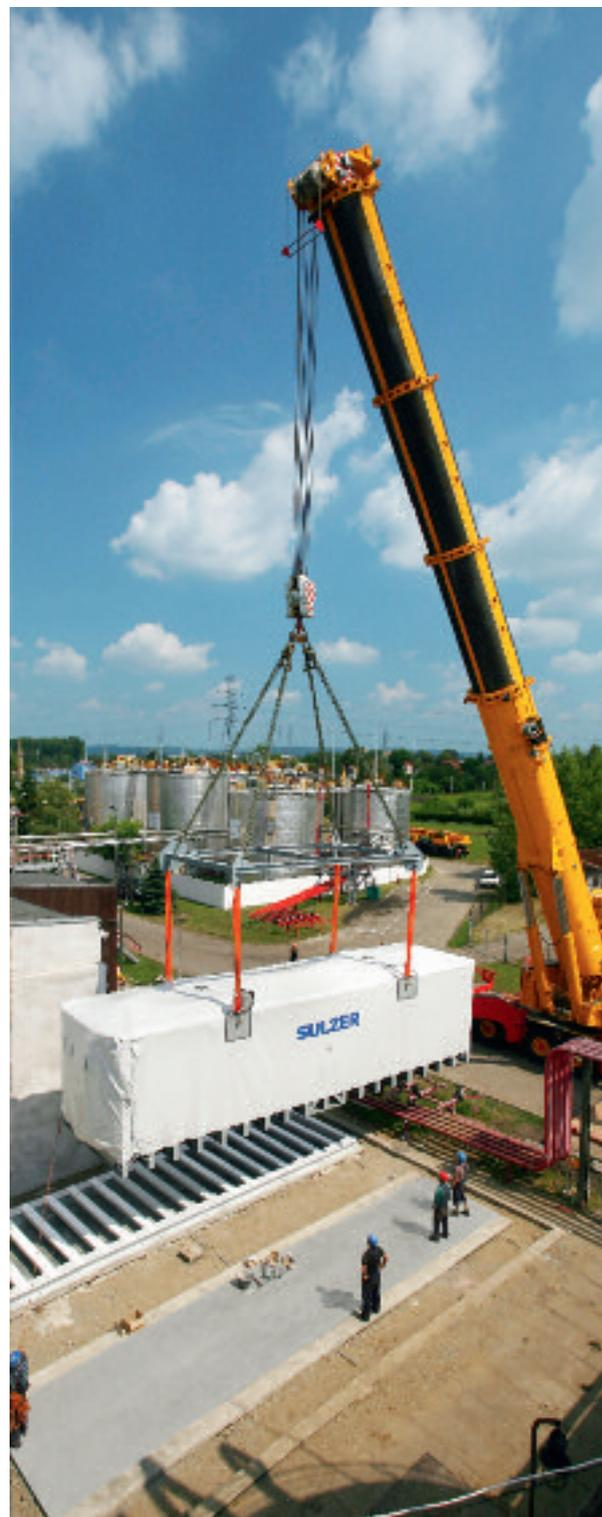
3 Sulzer installed a new paraffin deoiling plant at the Polish company Polwax.
