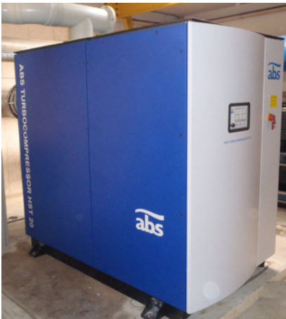
HST turbocompressor installation at Laon treatment plant in France
