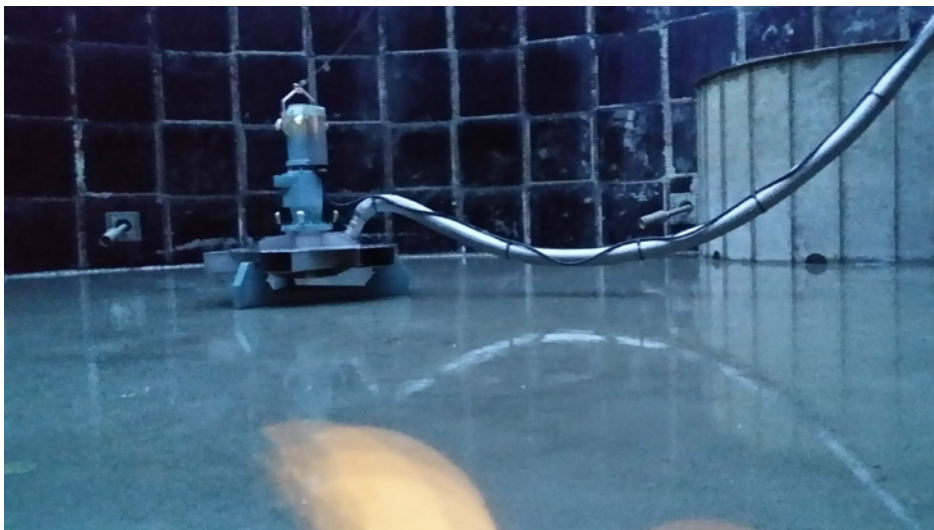
The OKI 2000 E-37AM with air hose at the bottom of a circular aeration tank.
