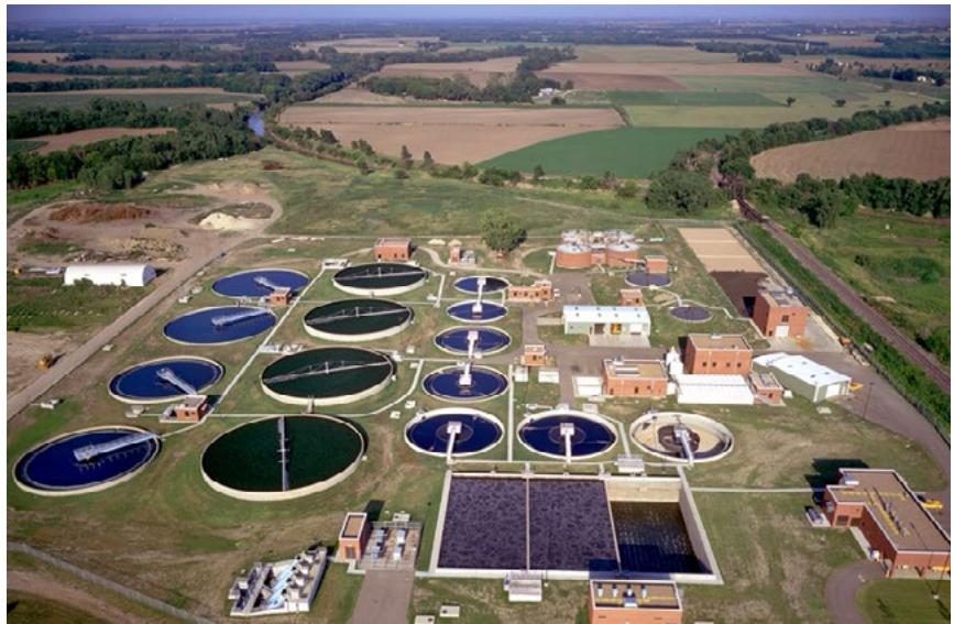
Salina's wastewater treatment plant
