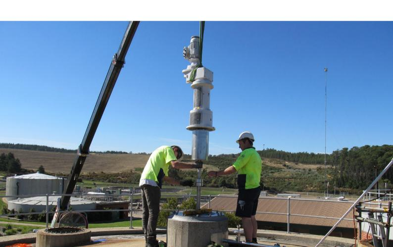
"Sulzer's highly efficient Scaba agitators are an optimum fit for sludge digestion. VFA (volatile fatty acids) decreased from 90% down to 65-70%. After the installation of the Scaba agitator, gas production has increased by 100%. Achieving this mixing energy with a 1.5 kW motor is remarkable."
