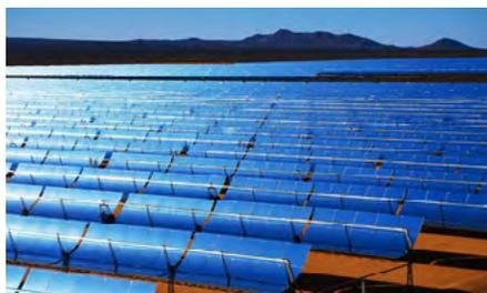
To promote renewable energy, the Chinese government has launched its first batch of 20 concentrated solar power (CSP) pilot projects using various technologies: central tower, parabolic trough, and linear Fresnel collector. Most projects will be equipped with a molten-salt heat storage system to last 6–15 hours. The Aksay plant is one of these 20 pilot projects.
