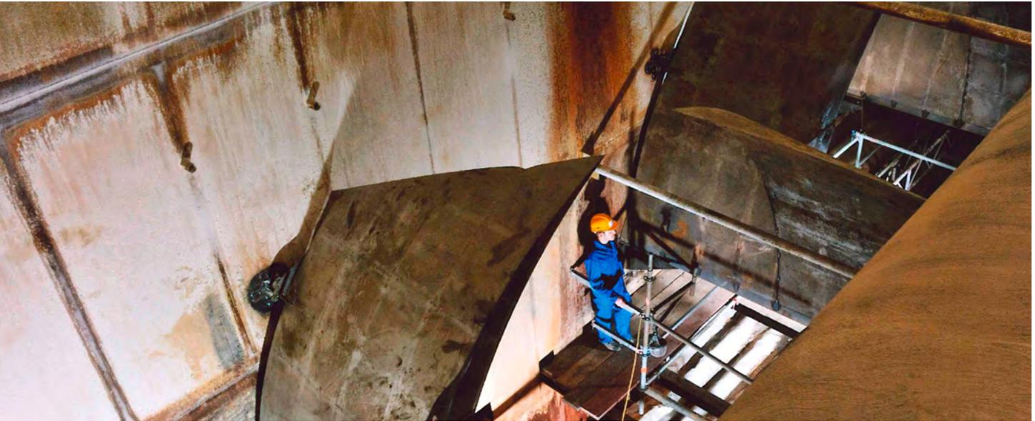
1 Installation of the Contour™ mixer from Sulzer into the flue gas duct of a power plant of GKM, Mannheim, Germany.
