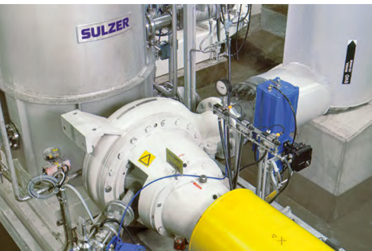
8 MCE pump with integrated degassing system.
