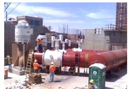
Installation of pumps and motors at the UP05 Project A expansion
