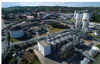
The Tereos Dobrovice plant with an integrated WWTP
