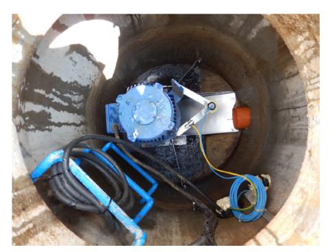
Sulzer engineers proposed an a Muffin Monster 10k low speed grinder and two Piranha grinder pumps which would use Sulzer's unique cutting technology to further reduce the solids, and generate the pressure required to transport the wastewater away from the site.
