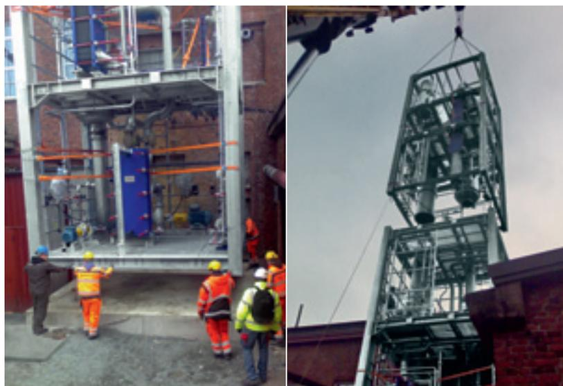
3 The installation of the plant's lower and upper skid sections at the customer's site in Finland required only minimal on-site activity due to the modular fabrication concept.
