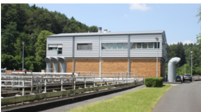
Compressor room behind the basin, intake manifolds for the aeration on the right side
