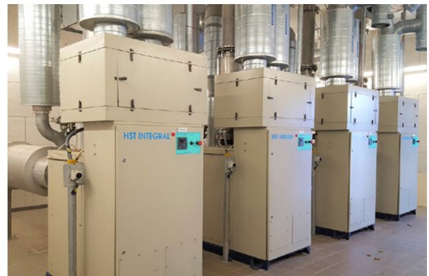
The original installation of four turbocompressors
