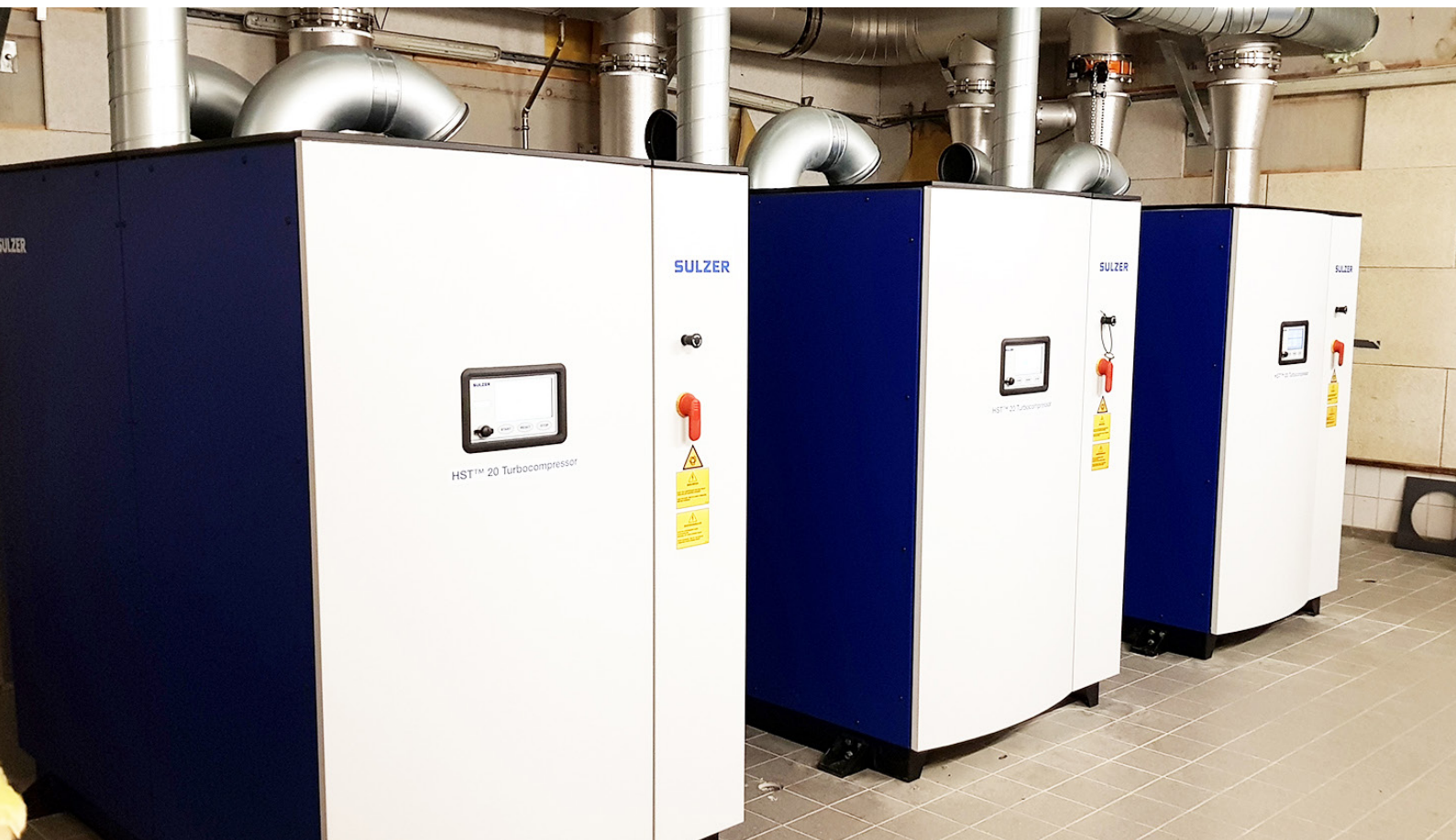
The new installation of three HST 20 units
