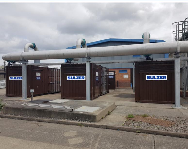
NWL's concerns with the poor reliability and rising running costs of their 20-year-old aeration blowers at Hendon STW meant a solution was needed. The terminal failure of one of these blowers in late 2019 caused the project to become critical. Sulzer were contacted and they installed a hire blower within three days which enabled the process to continue.
