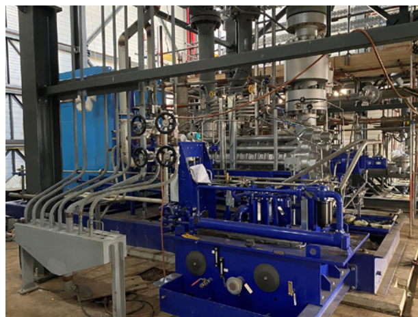
Site installation of feedwater pump
