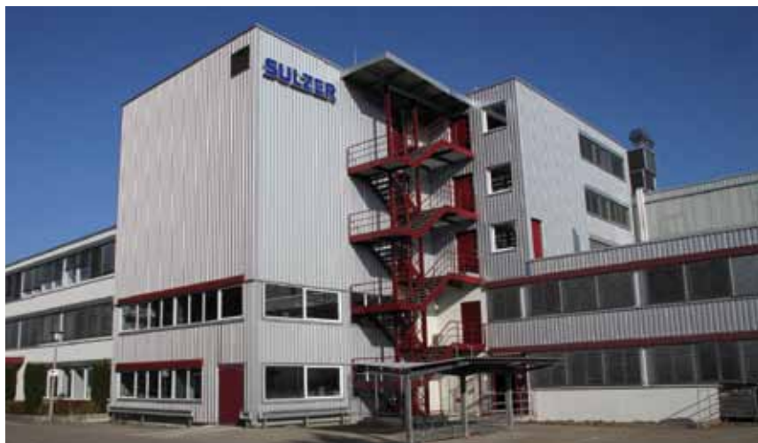
Sulzer test center in Allschwil, Switzerland
