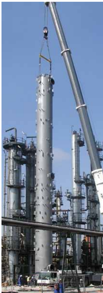
Installation of an industrial scale ECR extraction column
