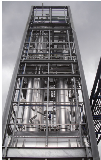
Skid-mounted unit with Pilot unit of an EvapCare™-F as column reboiler
