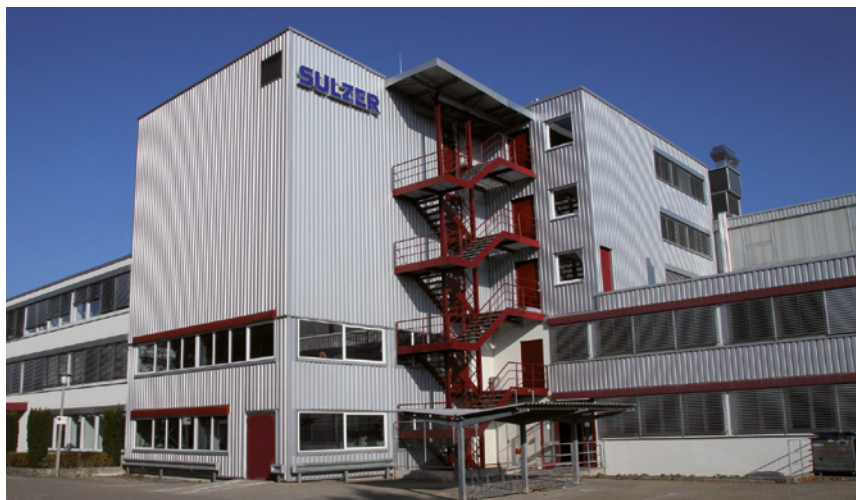
Sulzer test center in Allschwil, Switzerland
