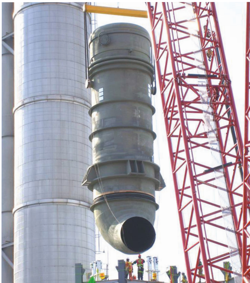
On-site installation of a large EvapCare™-F
