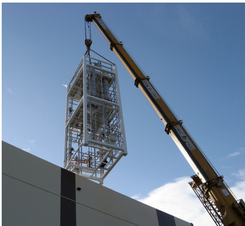
Two-stage skid-mounted evaporation unit with an EvapCare™-F and an EvapCare™-W
