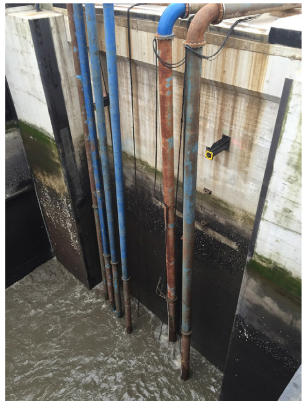
Rental pumps in the lock chamber: parallel installation of six flange pipes
