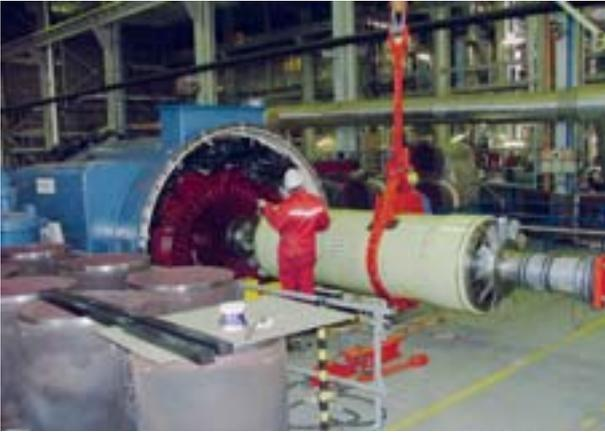
**4** Removal of the generator rotor.
